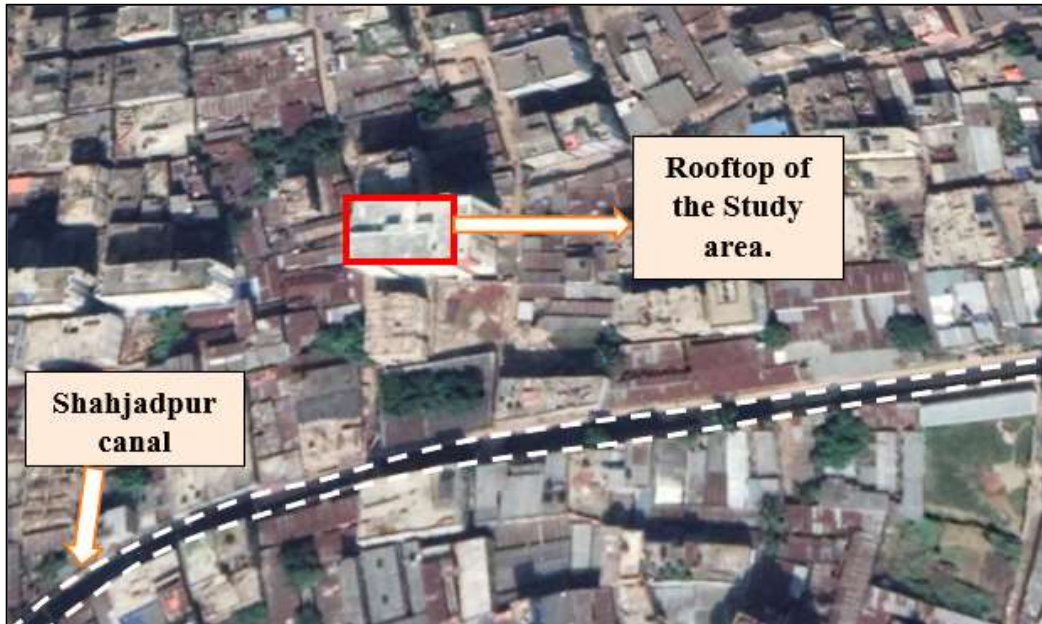
Figure 3: Aerial view of the study area. A 10 storied building with more than 33 meters in height which should be comprised of a fire sprinkler system in accordance with the building code.
